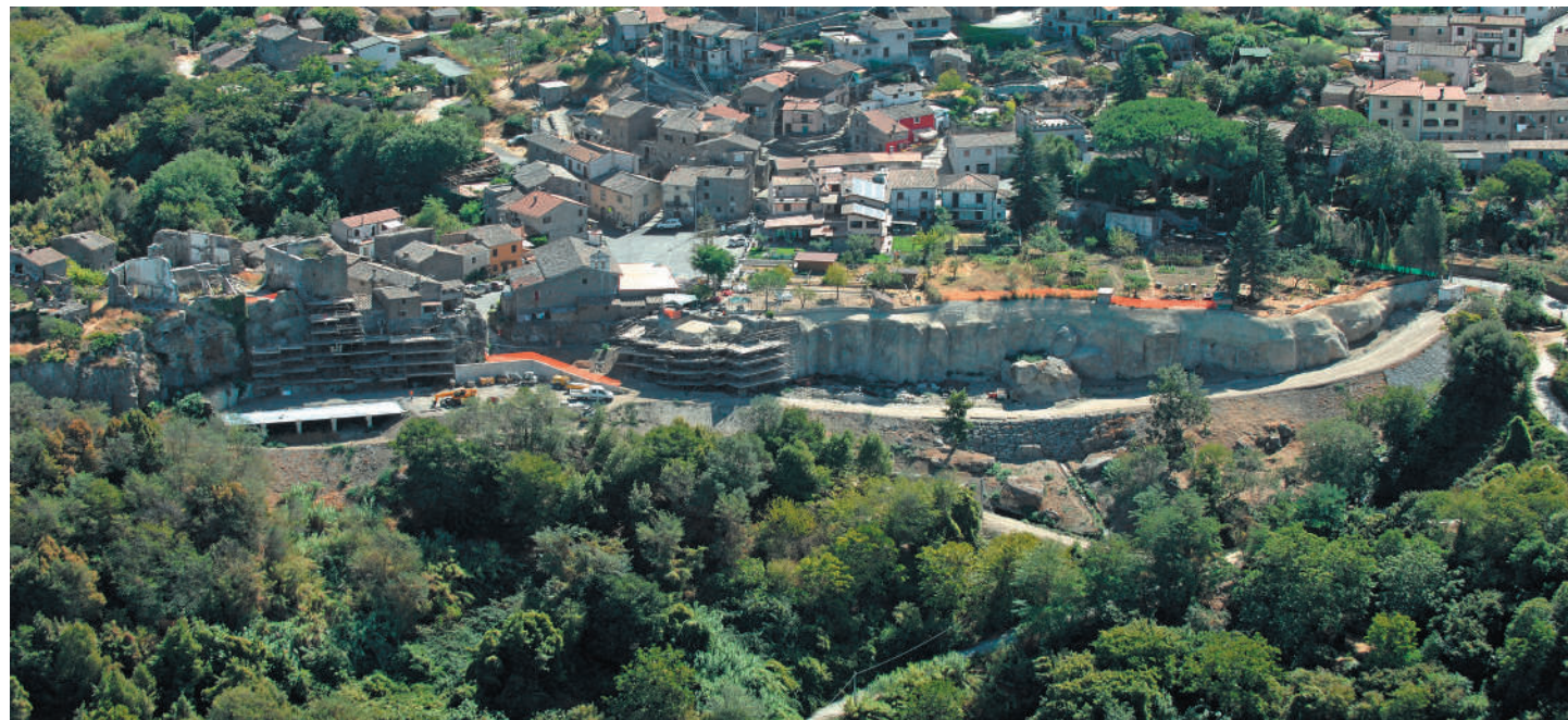
Ater Viterbo Consolidation, water regulation and safety of the crag in the municipality of Soriano in Cimino hamlet CHIA
