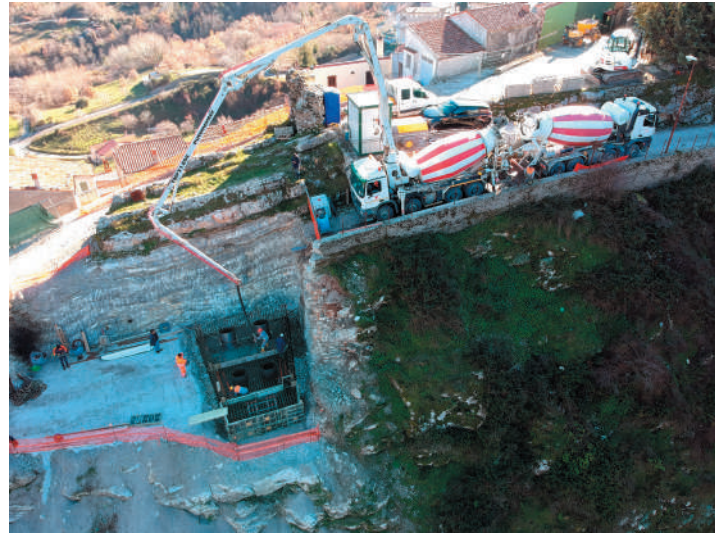
Work on the anchoring block of the bridge and the departure station
